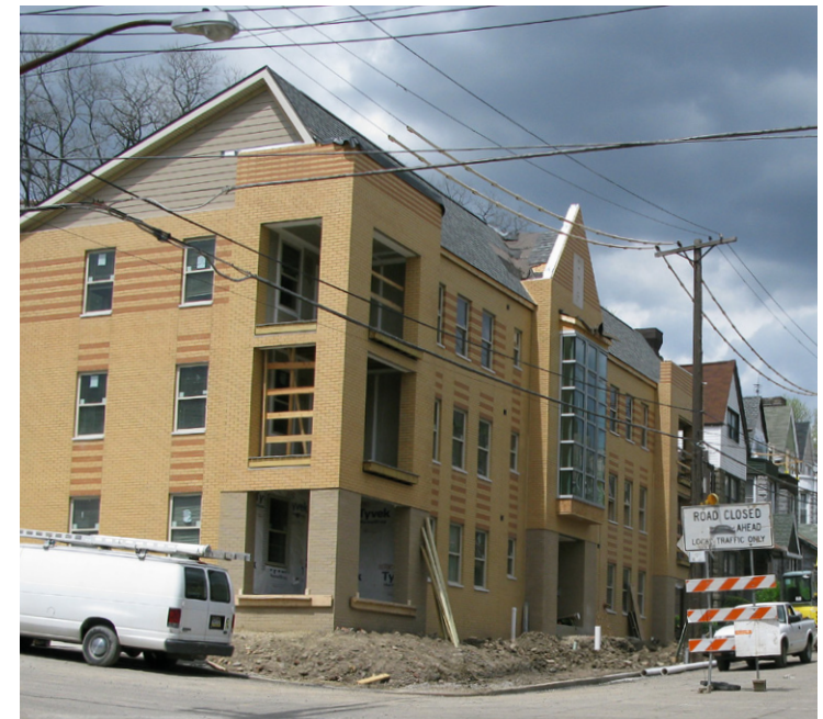
Residential construction in the Hill
