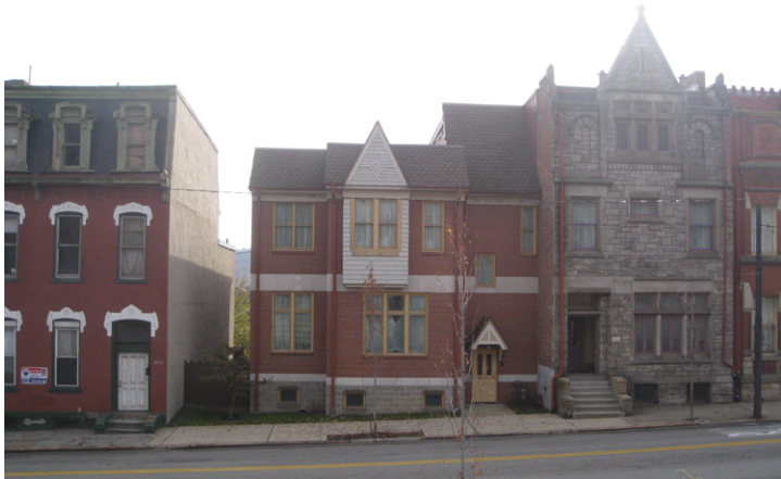
Existing residential infill in the Greater Hill District
