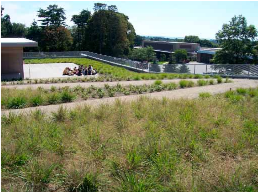
FIGURE 7.57 Above-ground retention
