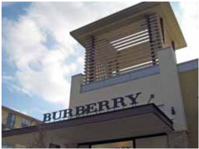
FIGURE 5.2 Example of signage projecting above onto a canopy [sect. 919.03.M7, (e)]
