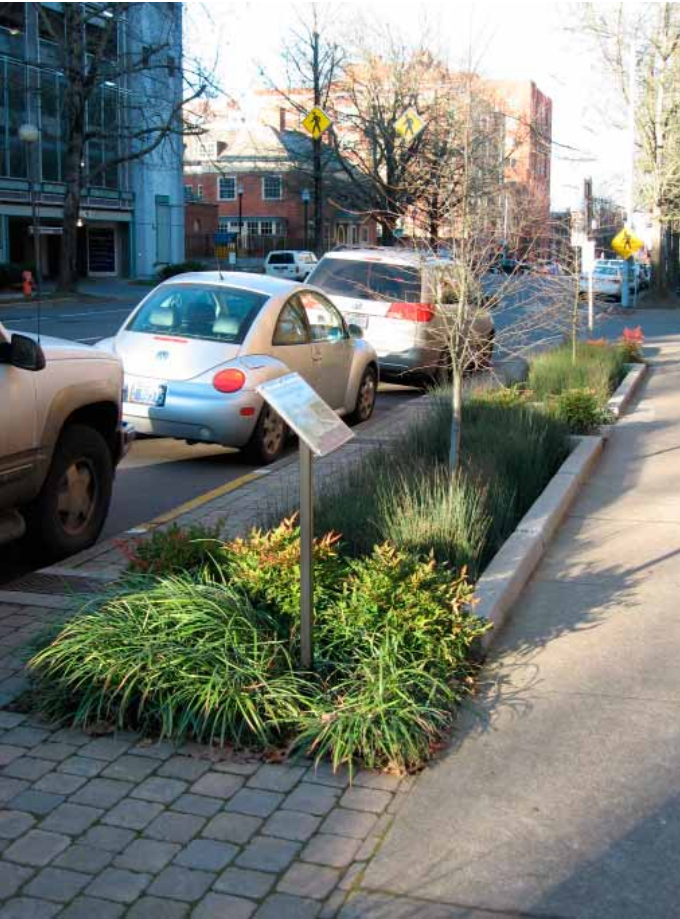
FIGURE 1.9 Example of a sustainable street design that contributes to reducing off-site runoff.
