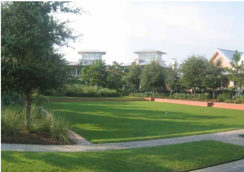
FIGURE 7.56 Passive stormwater retention occurs at this recessed lawn where rain can gradually infiltrate
