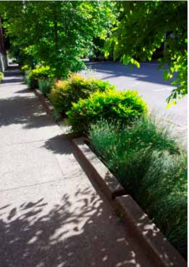
FIGURE 1.12 Curb cuts in planters allow stormwater runoff to enter infiltration planting pits.
