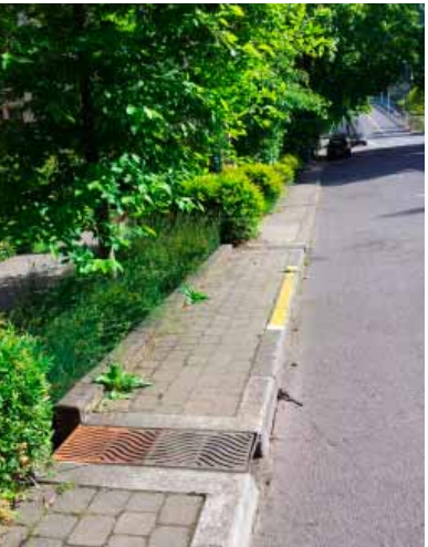
FIGURE 1.13 Decorative grates cover flush curbs allowing street runoff to enter infiltration planting pits.
