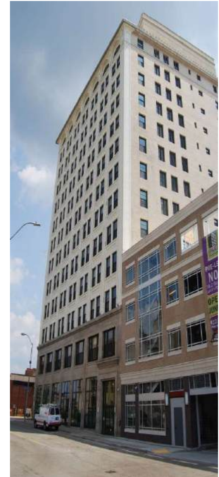
Highland Building Exterior
