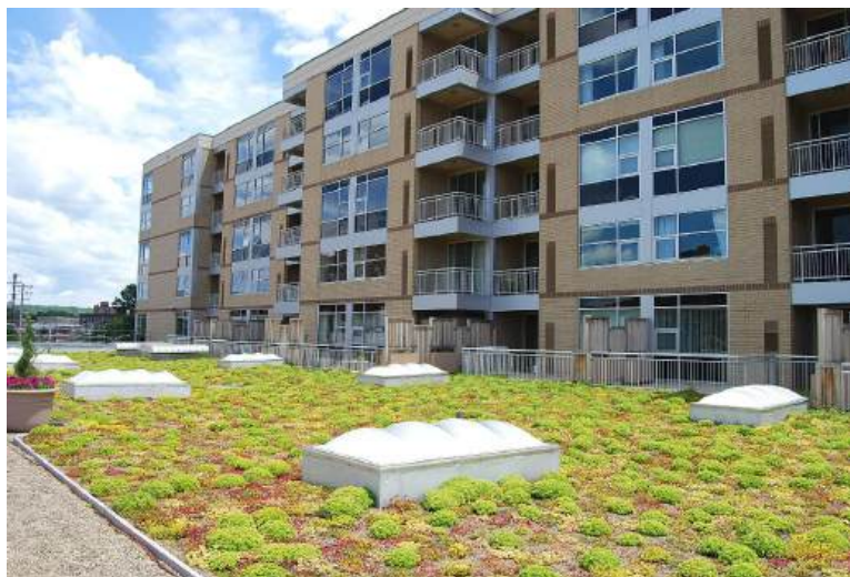
Market District - LEED Green Roof
