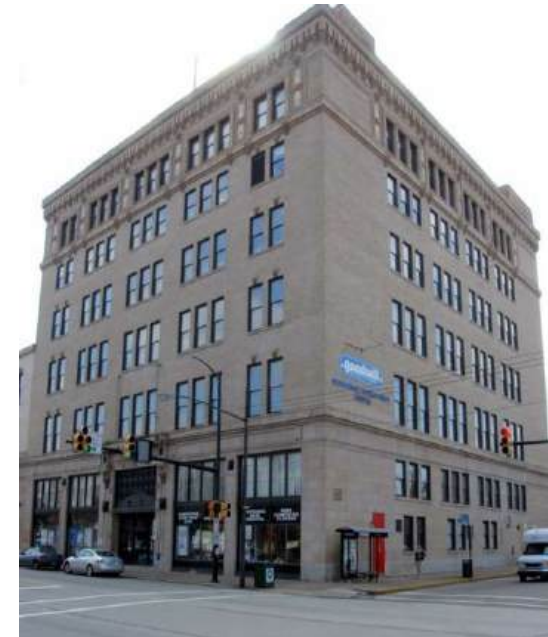
Brix Building Exterior
